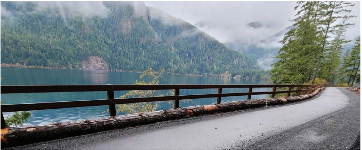
The Spruce Railroad Trail was recently reopened following construction. Photo courtesy Federal Lands Highway Division
